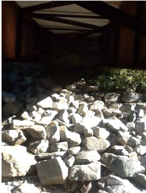
Left Bank Abutment when facing downstream
