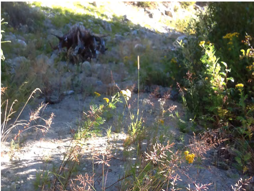
Left approach facing away from structure
