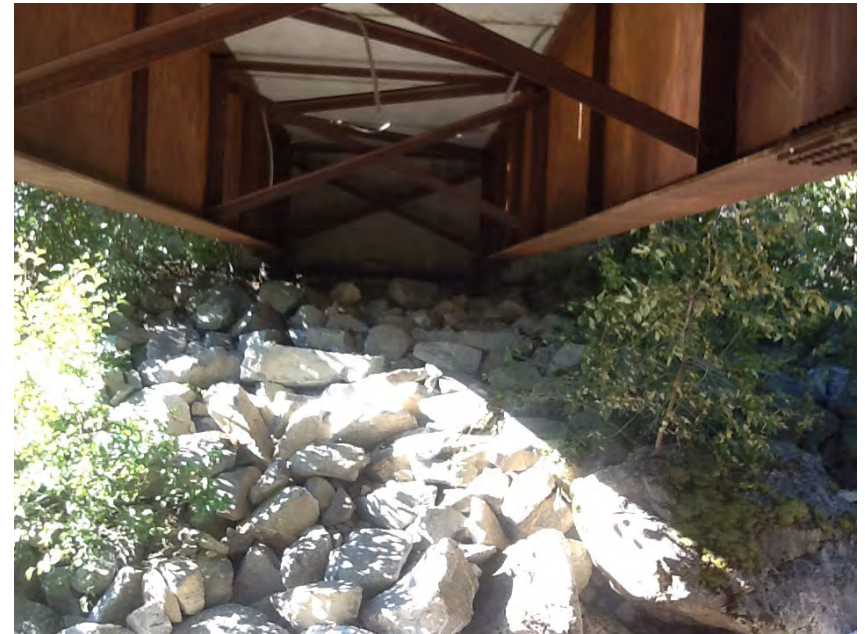
Right Bank Abutment when facing downstream
