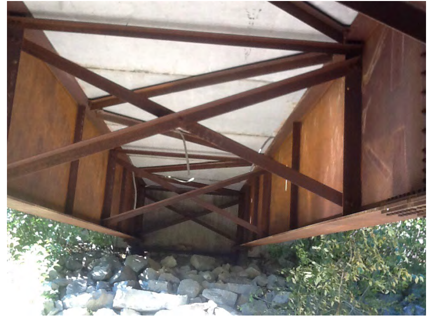
Underside of bridge
