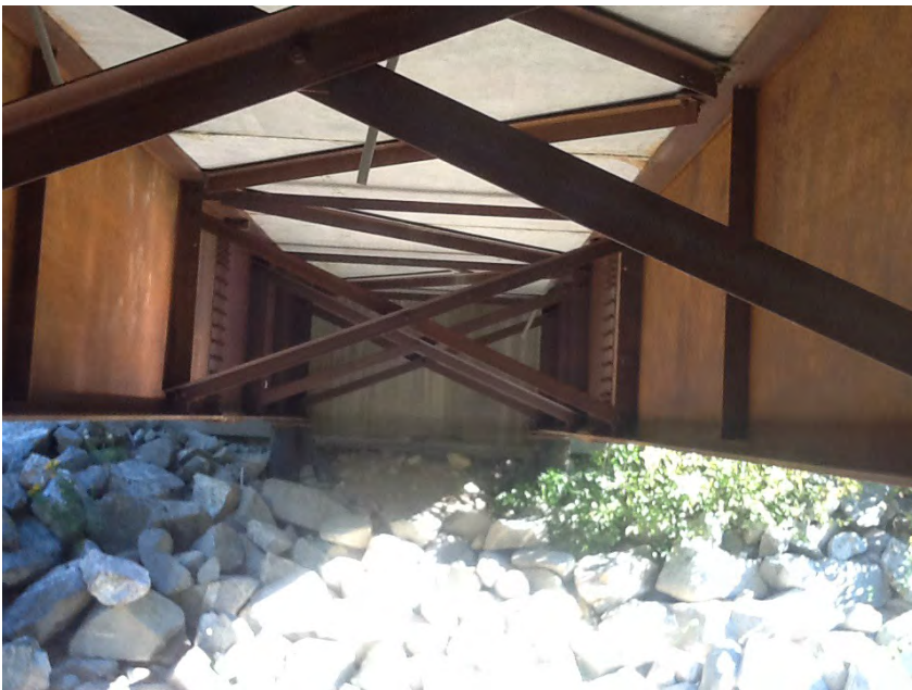
Left Bank Abutment when facing downstream
